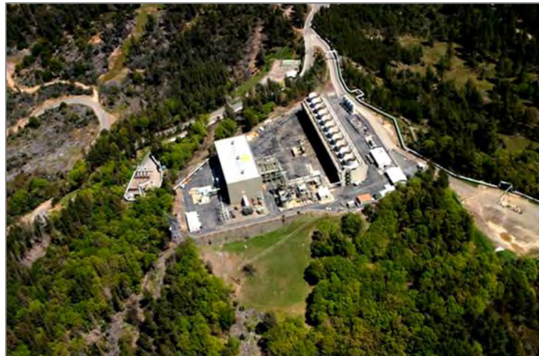
Photo 17-1, Cal Pine Generating Station at the Geysers
