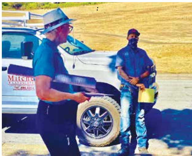
At last! Construction started in July on Oakmont's own dog park. Iris Harrell, Oakmont Building Construction Committee chair, confers with contractor Owen Mitchell beside Stone Bridge Road as Mitchell prepares to start the two-month job of creating the park. (Photo by Julie Kiil)
