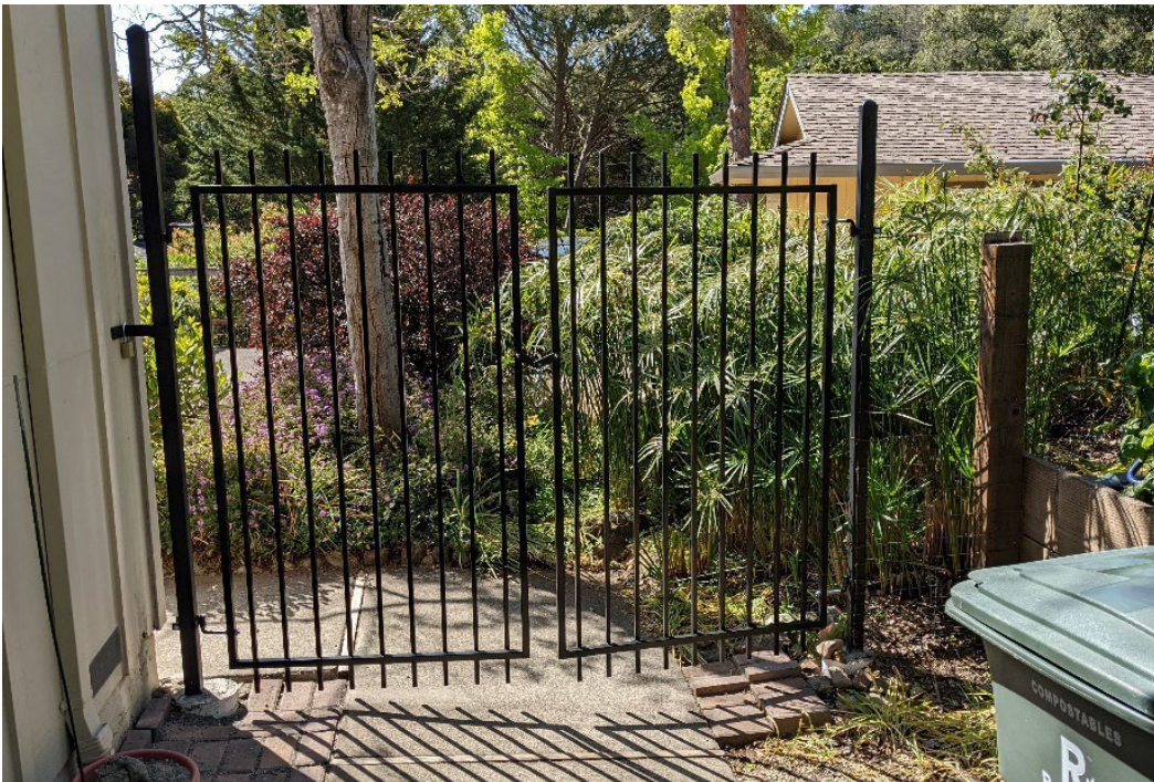
Gate #6 Type 17 - Stock sized gates & hardware ordered from one of the local major hardware chain stores, installed by homeowner.
