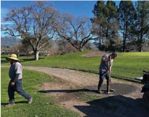
The maintenance crew fills in potholes at Valley of the Moon golf club's hole 17. The team has been busy filling all weather-created potholes on the cart paths at both Valley of the Moon and Sugarloaf golf clubs. (Photo courtesy of Valley of the Moon Club Facebook page)
