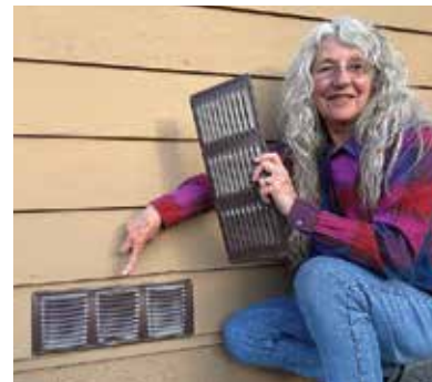
Pre-Vent embers with 1/8" metal screen (this one has lowered cover). (Photo by Louisa Knabe)
