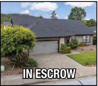
5992 Stone Bridge Road
